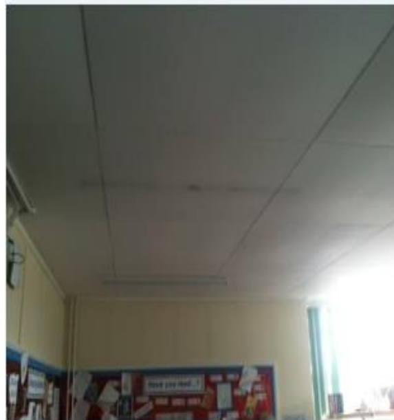
Shows gap where old light removed
